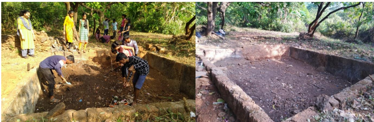
Compost Pit after completion of work
