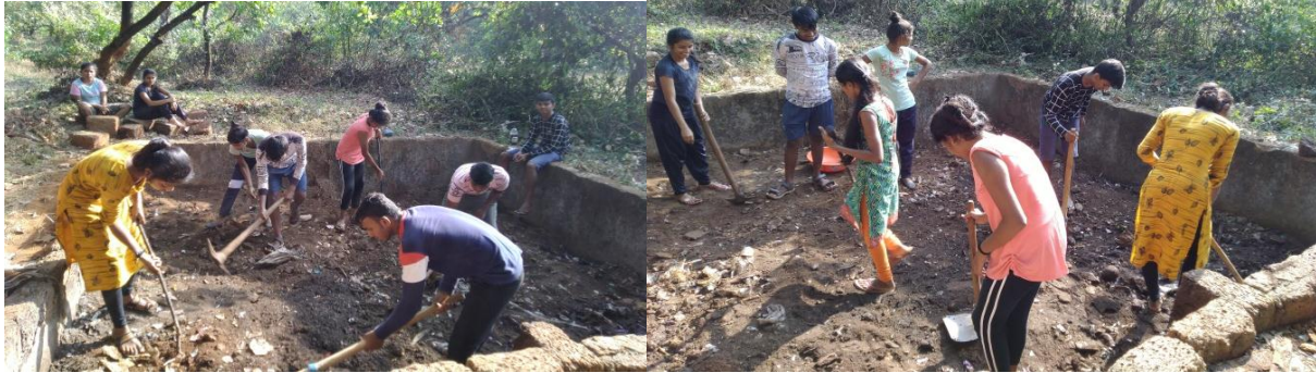
Cleaning & digging of Compost Pit in progress
