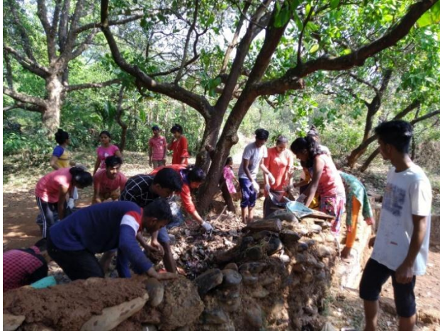
Construction Work In Progress
