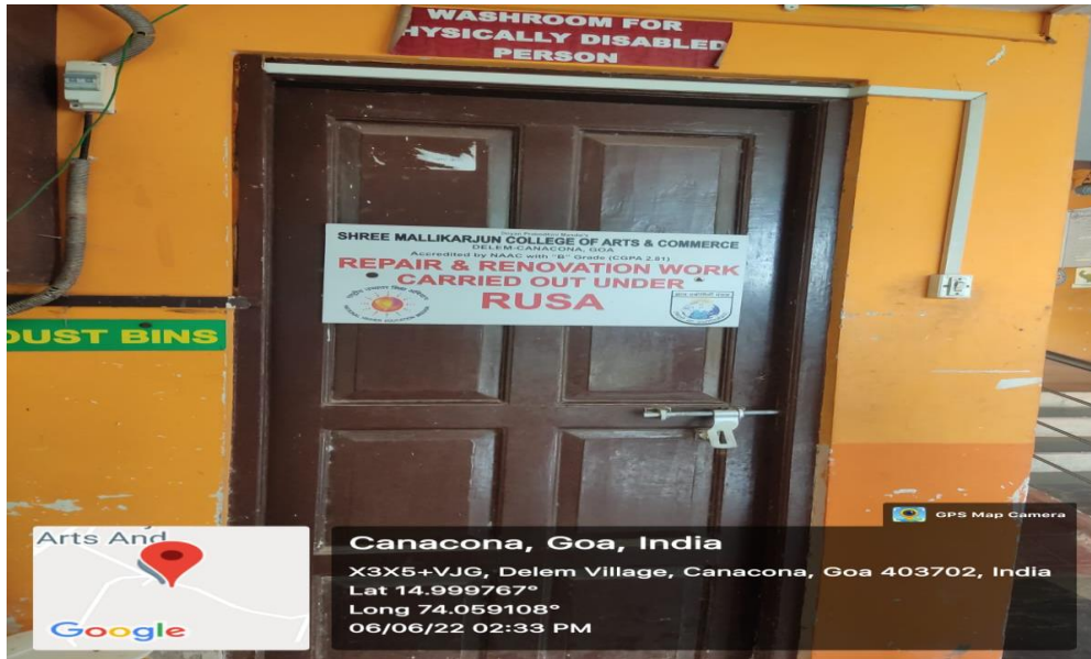
WASHROOM FOR PHYSICAL DISABLE
